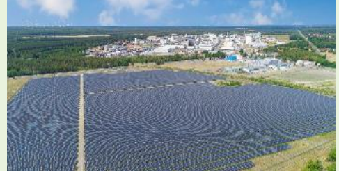
On-site solar park Schwarzheide, Germany
